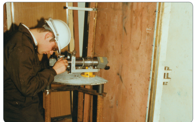
Checking a watertight seal on the bulkhead
