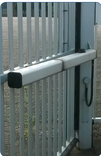
Figure 3 - Lead screw application in automatic gate
